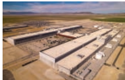
Facebook Data Center 970,000 sq ft building $1 billion project
