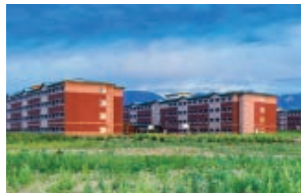
Fort Carson 13th CAB Barracks 486 blast resistant wall panels 226,000 sq ft
